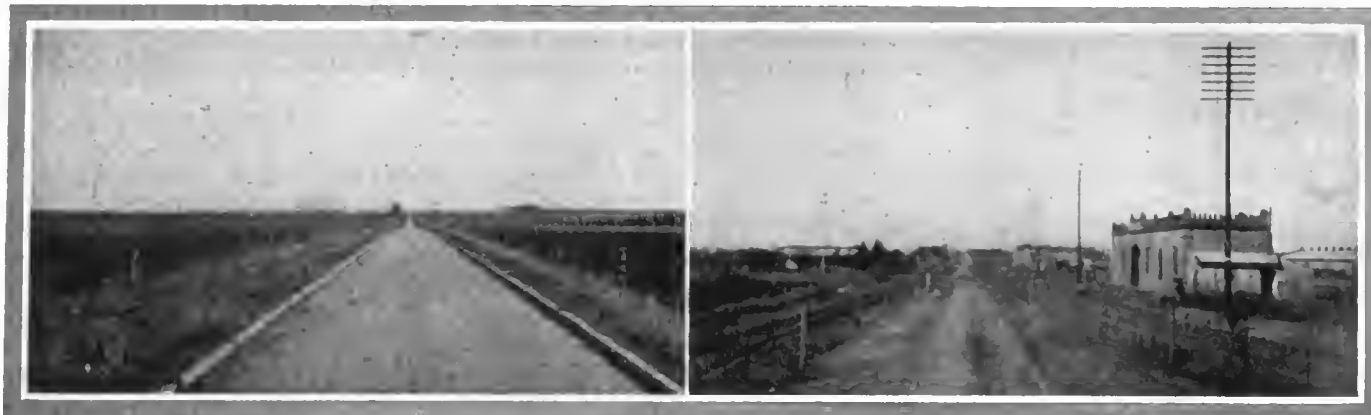
Left—There are 63 miles of this stone block road between Buenos Aires and La Plata. It is Argentine's finest road. Right—Touring road between Buenos Aires and La Plata, which is built in the middle of the dirt wagon road
